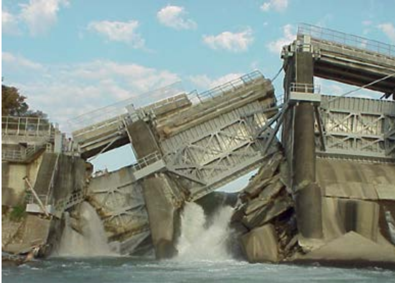
↑ Figura 5. Daños de presa Shih-Kang después del sismo de Chi-Chi (tomada de Observed Performance of Dams During Earthquakes (p. 10), por Tim Little, 2000, U. S. Committee on Large Dams).
